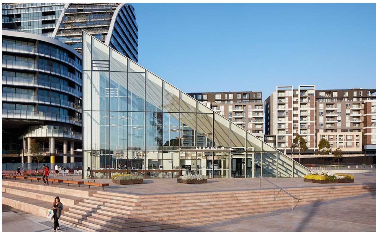
Figure 3 Green Square Library – community infrastructure for the growing population
